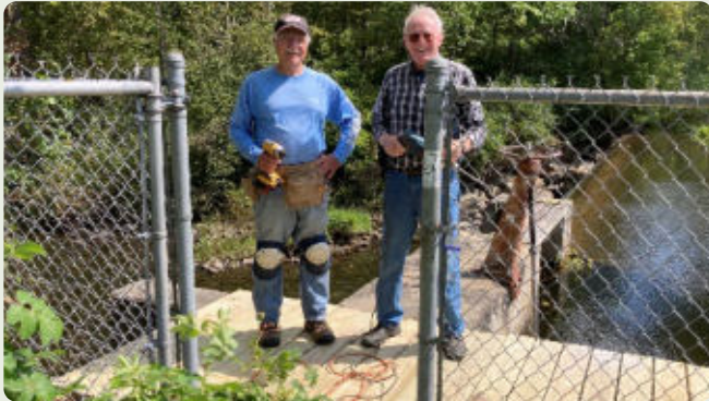
Dam Committee Members Complete Decking
